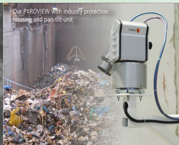
Hot spot in a waste bunker
